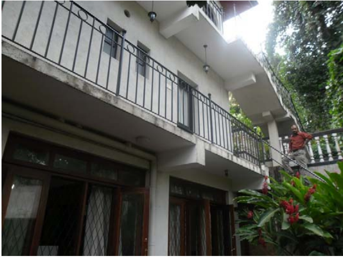
Second floor side entrance to the apartment
