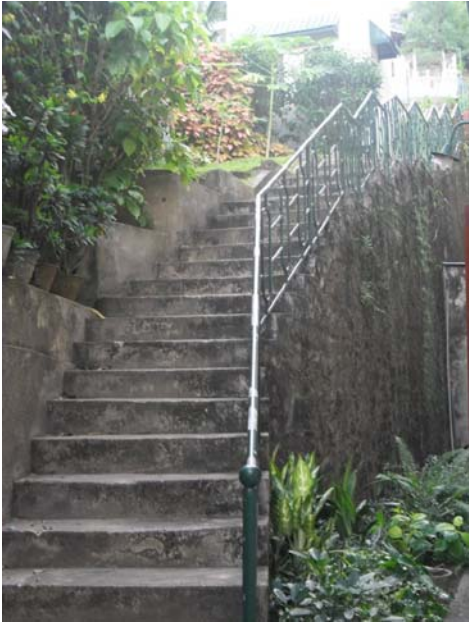
Stairway from the main entrance to the apartment
